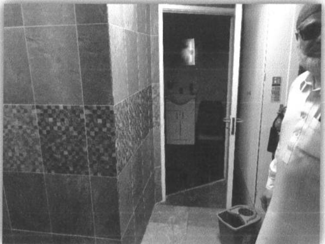
Image of the accessible toilet.
